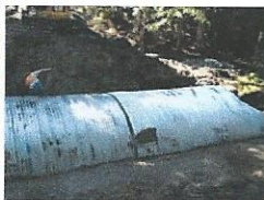
PUD CULVERT REPLACEMENT
